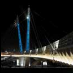
SHA LU OVERPASS Taiwan
