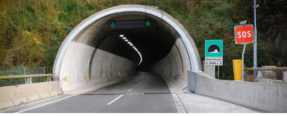
Fael LUCE, thanks to the experience and know-how acquired in the **high-power professional lighting sector**, has been able to solve very well the visual task required by the Customer with the new, innovative and advanced series of luminaires for ARCALED tunnel lighting.
