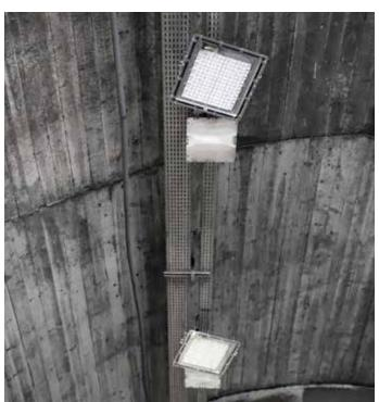
The **EASY FIX** system, designed for the adjustment of the lighting device, has allowed the rapid and precise installation of the luminaire on the channel placed, in this precise project, is located in a decentralized position with respect to the center of the roadway, ensuring perfect adaptability to the most heterogeneous road layout within the same tunnel.
